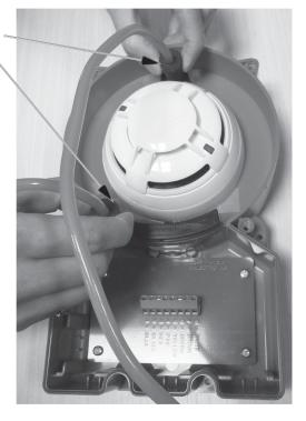
6 ONCE THE MEASUREMENTS ARE TAKEN, SET ASIDE THE MANOMETER, REMOVE BOTH RUBBER GASKETS, REINSTALL THE DIVERTER, AND CLOSE THE LID WITH THE SCREWS.
